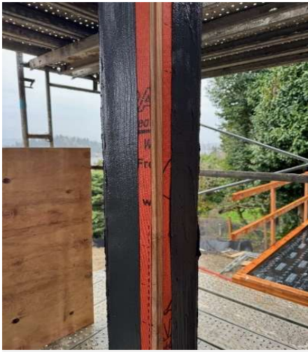
orange and black waterproofing products applied to a stud
