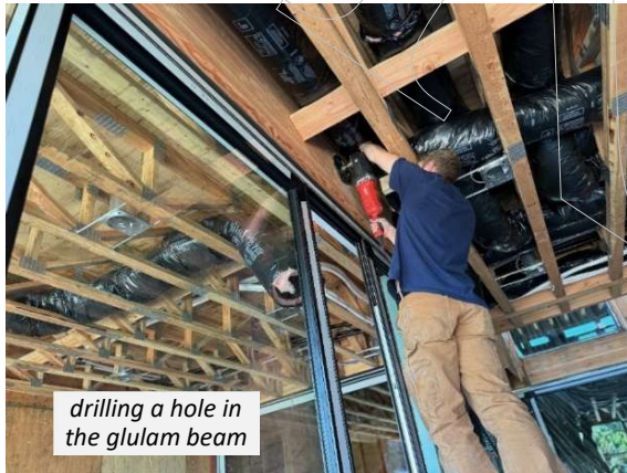
duct passes through glulam
