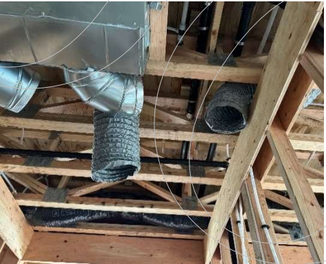
ceiling return air outside Mechanical Room door – centering it meant having a beam in the middle (will be hidden by register)
