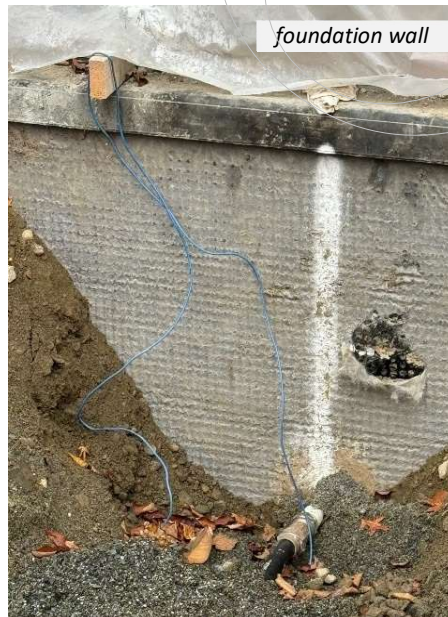
pipe from Playroom exits foundation wall and connects to black pex running to water meter
