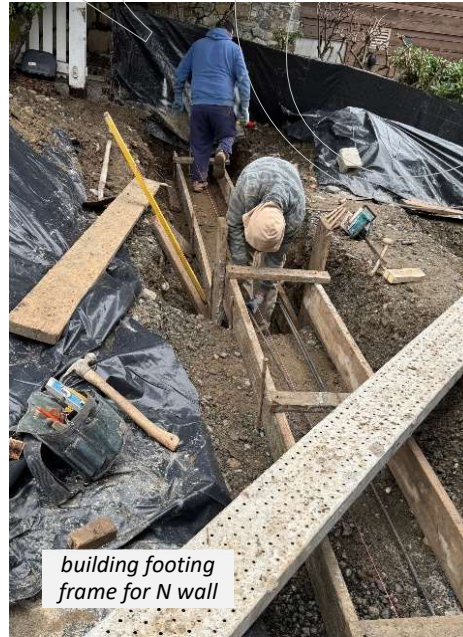
building footing frame for N platform
