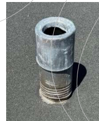
example of a roof plumbing vent
