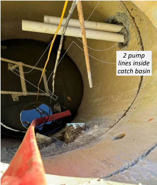
trench on S side with 2 pump lines
