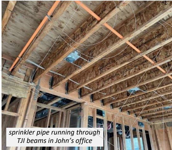
sprinkler pipe running through TJI beams of Great Room
