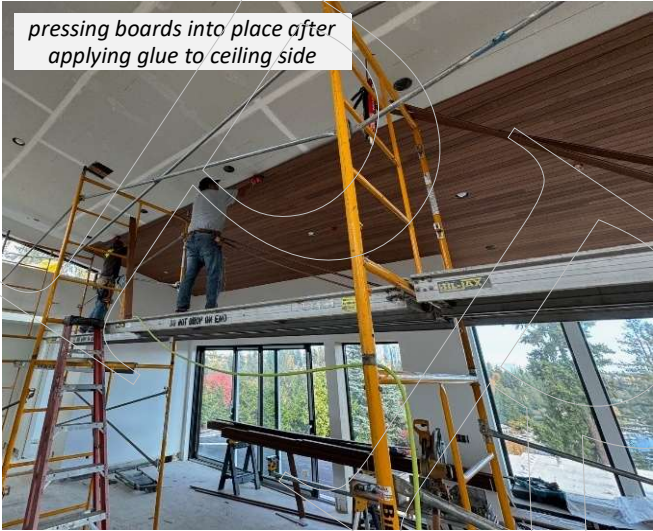
heavy duty adhesive used to glue wood panels to ceiling
