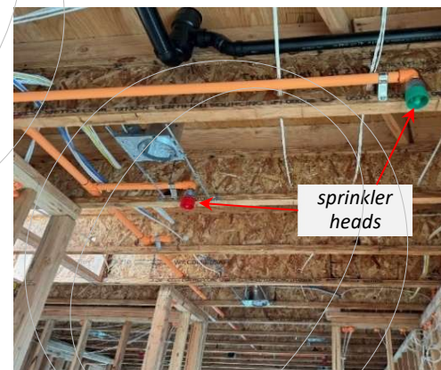
fusible link sprinkler head with deflector extended
