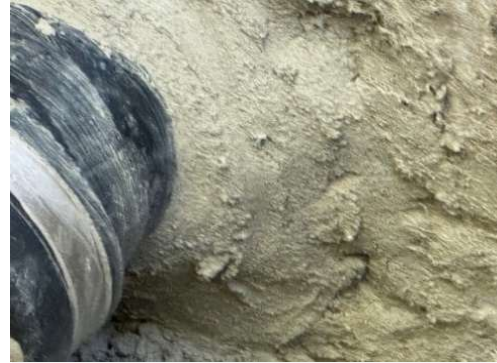
after covering with a sealant
