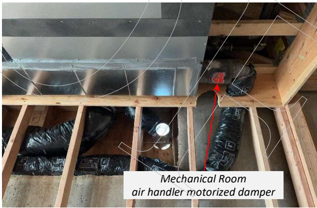
motorized dampers
