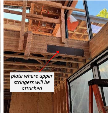
temporary platform built to support the landing
