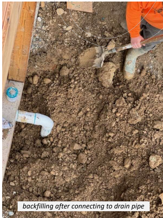
covering the PVC pipe in the Atrium
