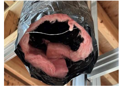
flexible supply ductwork with insulation
