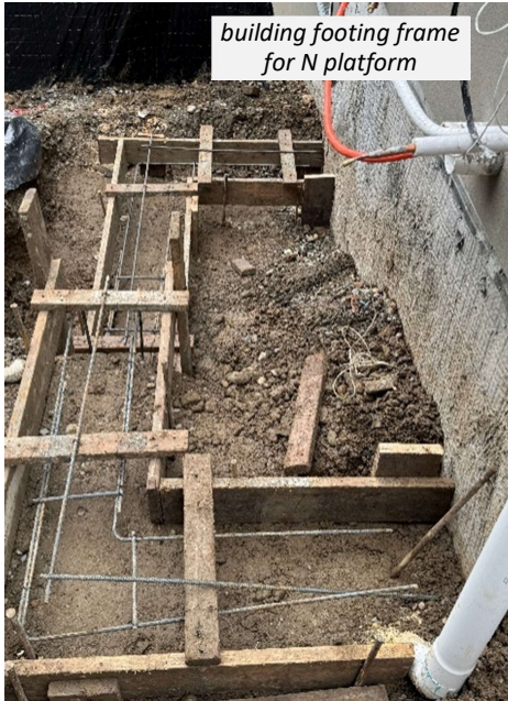
building footing frame for N wall
