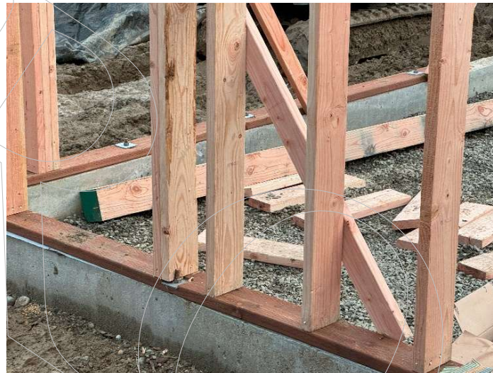
horizontal beam bolted to foundation wall
