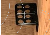
home run helper attached to joist
