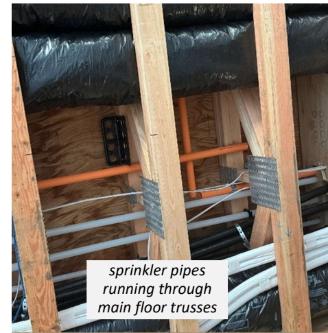
sprinkler pipe running through studs
