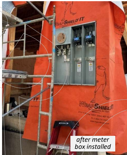
after Generac transfer switches installed
