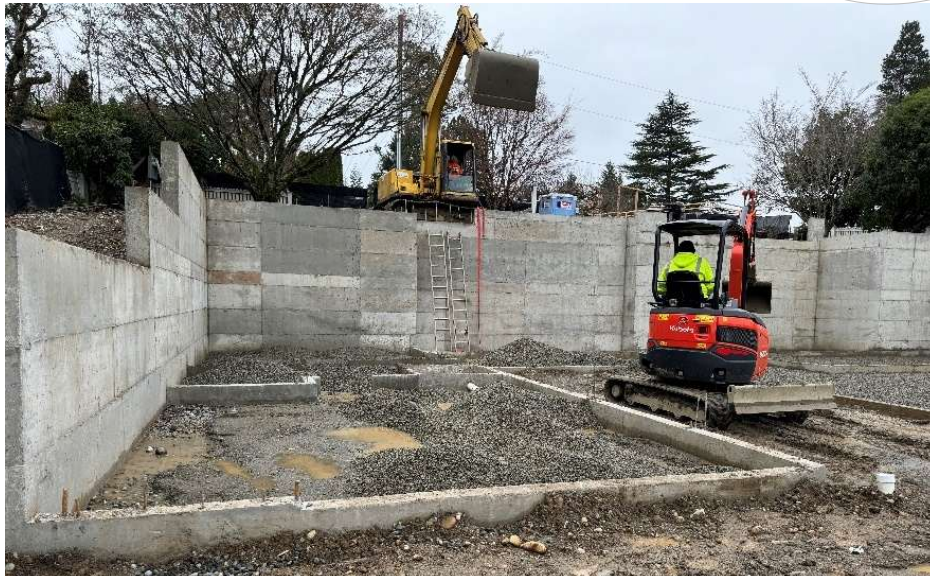
bird's-eye view Dec 1 before foundation filled with gravel burrow and crushed rock fill
