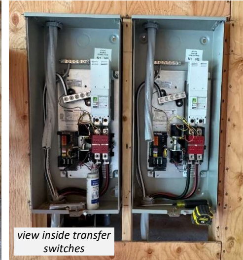
after Generac transfer switches installed
