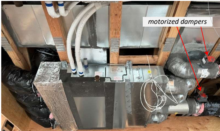
extending the rectangular air duct then creating forks to feed fresh air to air handlers
