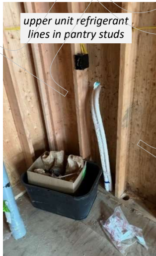
holes in N wall for upper and lower unit refrigerant lines
