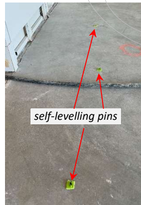
self-levelling pin after being cut
