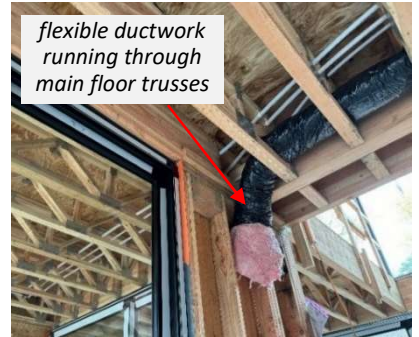
flexible supply ductwork with insulation
