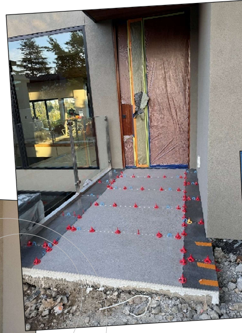
using shims for spacing
