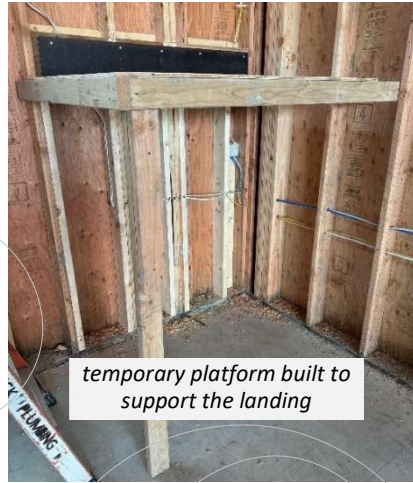
plate where upper stringers will be attached
