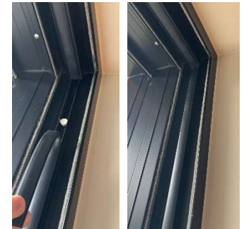
door open detector hidden under rubber strip
