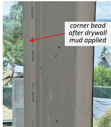
corner bead L shape metal corner with tape
