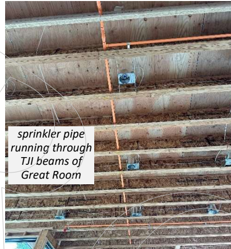
sprinkler pipe running through studs
